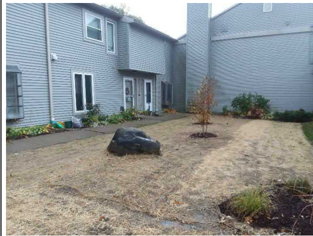
The drainage associated with the courtyard between Units 355-361 and 363-369 has been completed and the lawn areas seeded and mulched.
