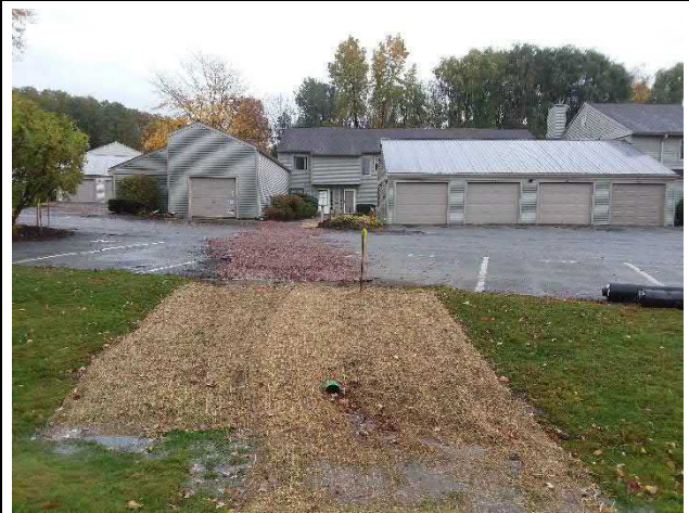
This new 6" PVC drainage pipe has been installed. The area surrounding the outlet has been graded, seeded, and mulched.
