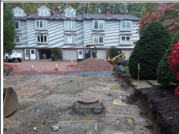
Subbase has begun to be laid down starting in front of Units 262-276.
