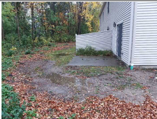
Ponding on the eastern side of Units 190-196 in the rear of the building.
