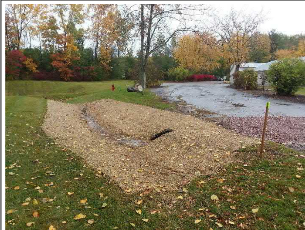
Newly installed 12" HDPE culvert near Units 411-417. The swale has been installed, graded, seeded, and mulched.
