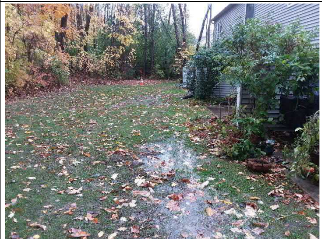
Ponding behind Units 170-176 in the rear of the building.
