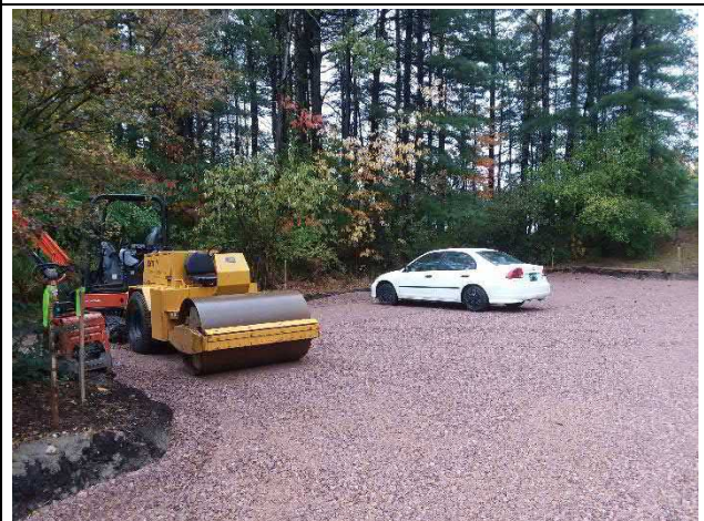
The subbase has been laid down in the parking spaces across from Units 262-276.
