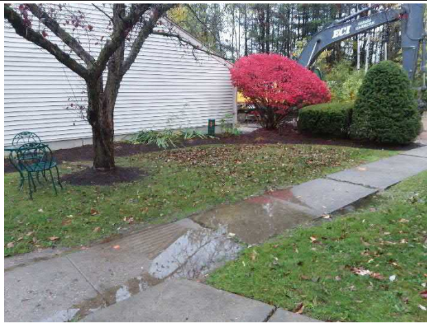
Ponding on the sidewalk in front of Units 281-287
